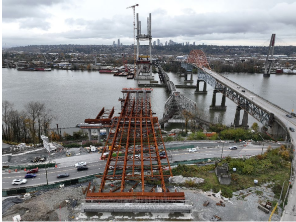
Figure 1: North Approach girder erection continues above Front Street in New Westminster.
