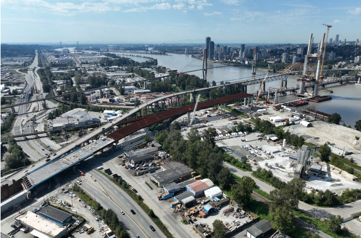
Figure 1 – In Surrey, bridge deck construction including deck panel installation continues.
