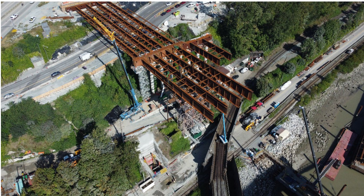
Figure 2 – North approach girder erection continued above Front Street in New Westminster.
