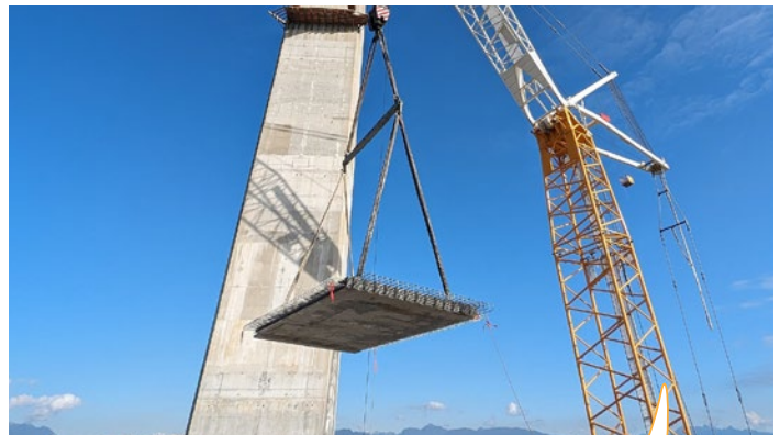
A concrete panel is lifted onto the deck.
