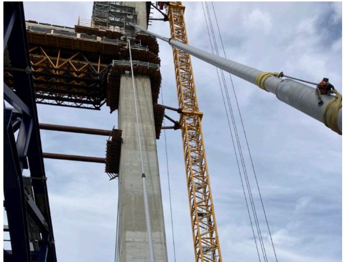
A view of the upper cable anchorages on the bridge tower.
