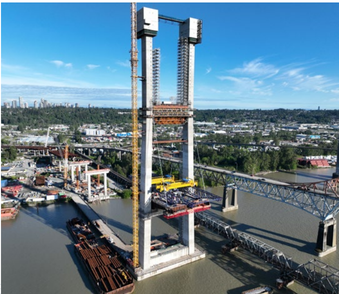
The bridge tower supports the bridge deck. Here, you can see the bridge deck starting to take shape.
