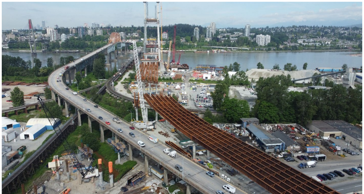
Figure 4 – Aerial of the south approach girder installation in Surrey.
