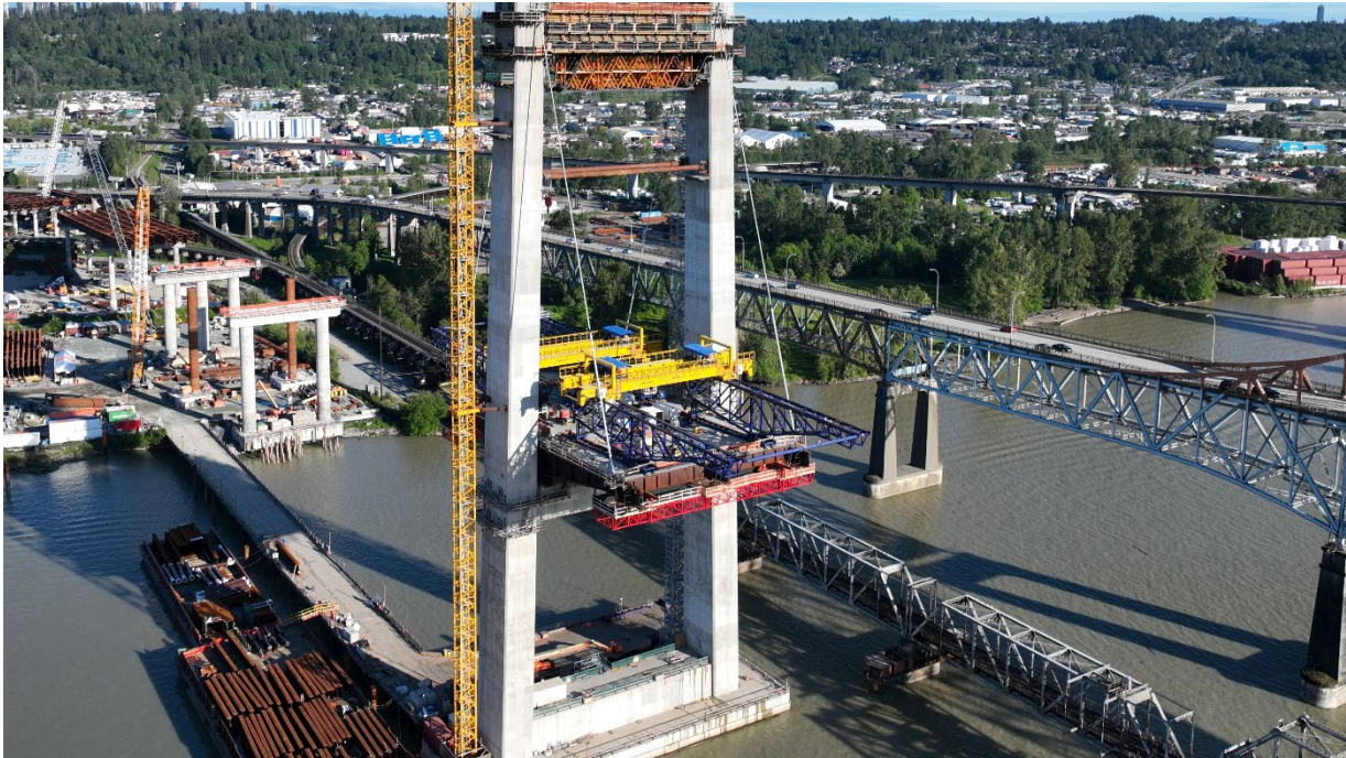
Figure 2 – Bridge deck construction continues.
