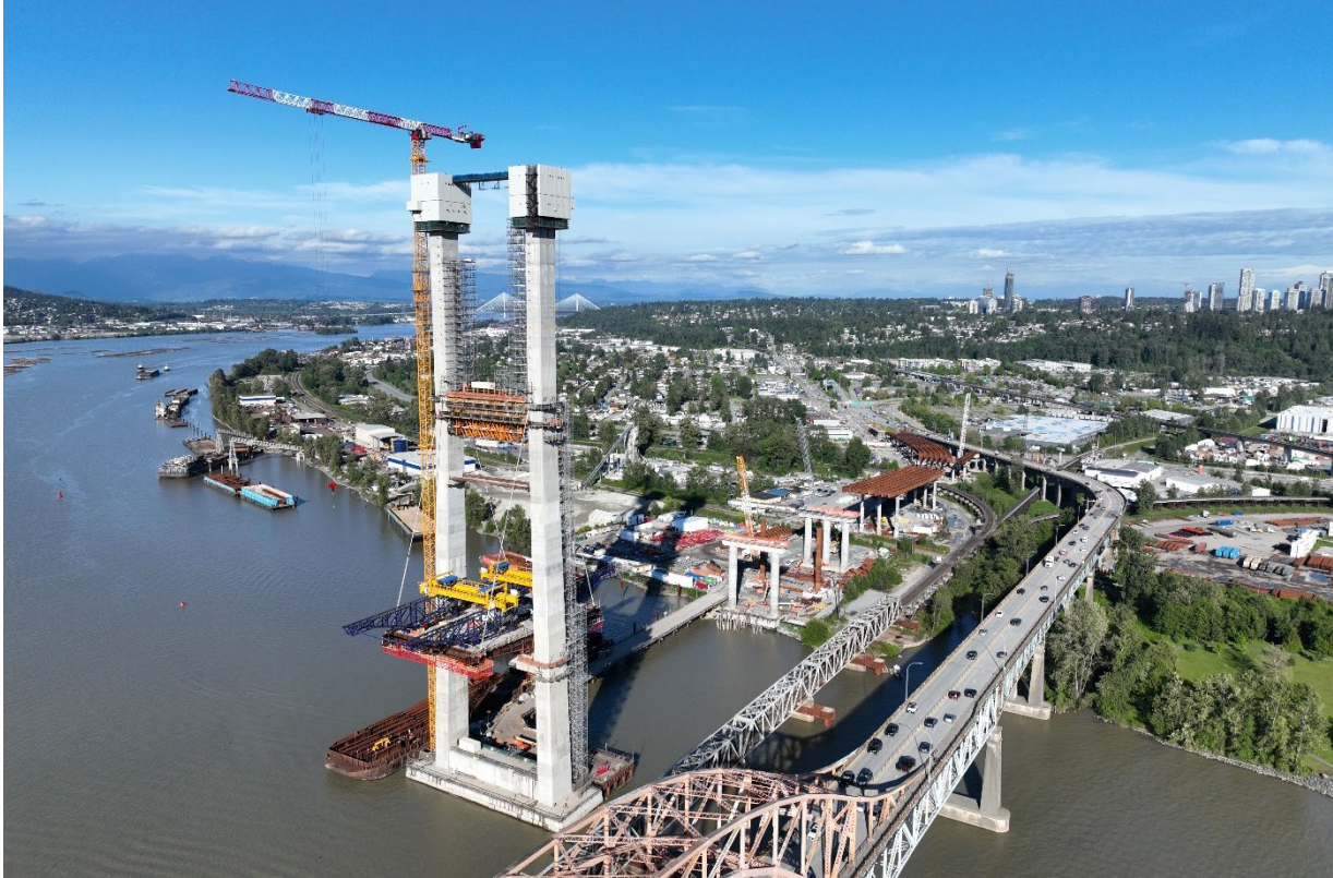
Figure 1 – Aerial of completed bridge tower.
