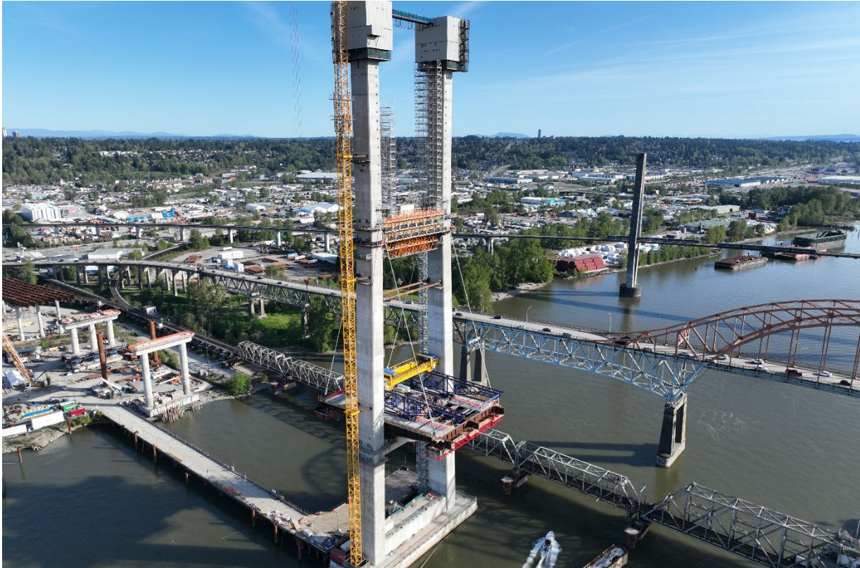
Figure 1 – Aerial of ongoing bridge tower construction.
